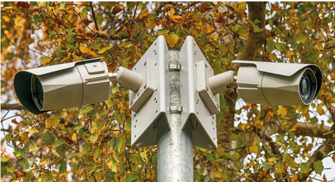
CCTV could act as a deterrent
